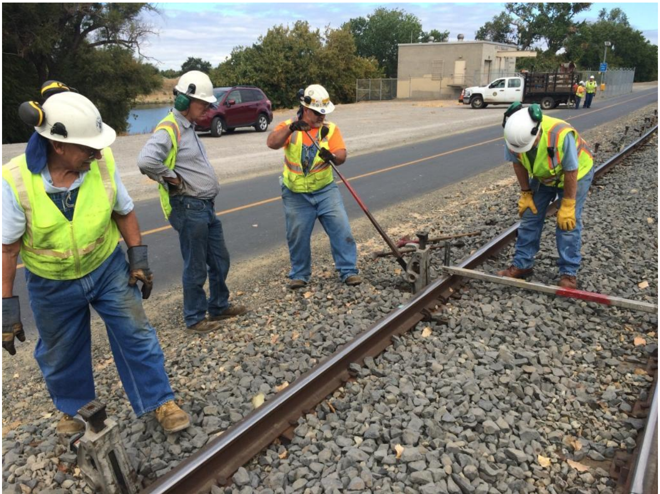
Mike F. lifts the west rail as Mike W. checks the level. Clem and Steve get ready for the next jack
