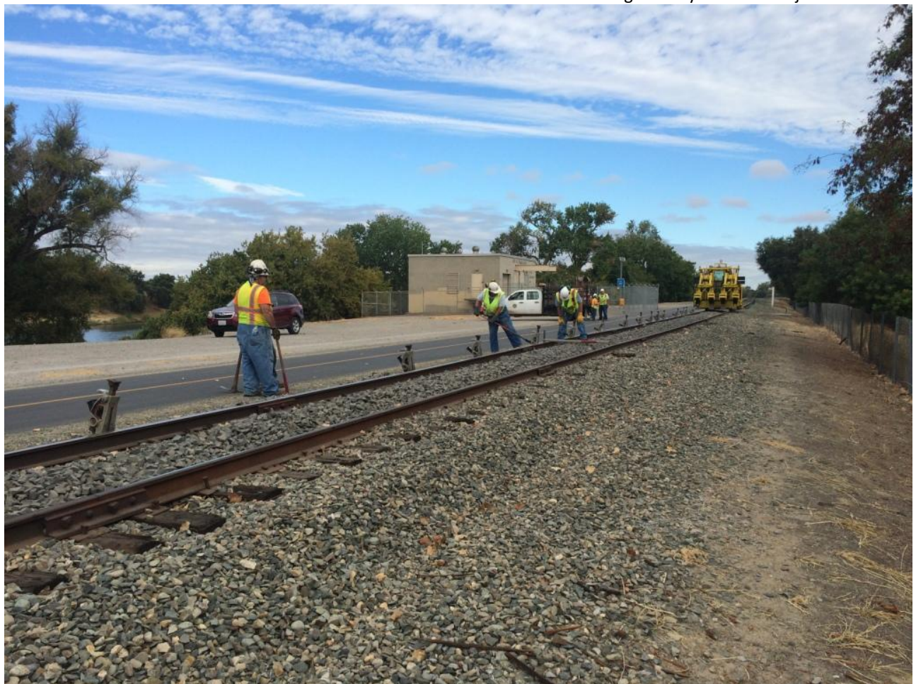
Jacks set, leveling in progress, bring in the tamper
