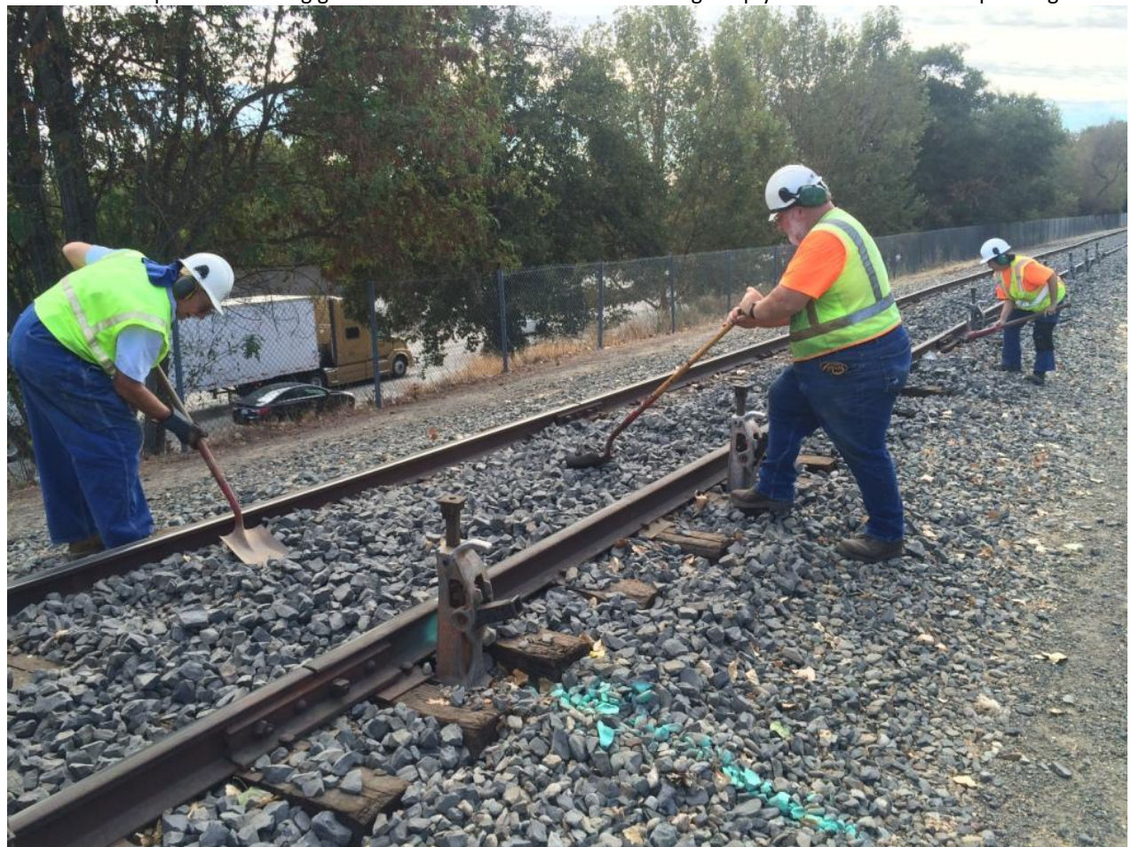
Clem, Frank, and Pam shifting ballast-rock so that there would be plenty for the tamper to shove under the ties
