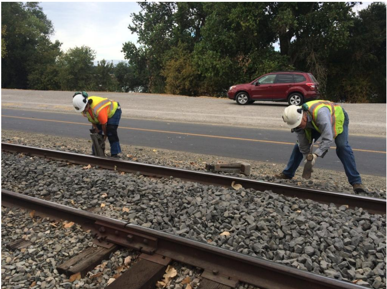
Pam sets a jack as Steve digs out a space for a jack to be placed
