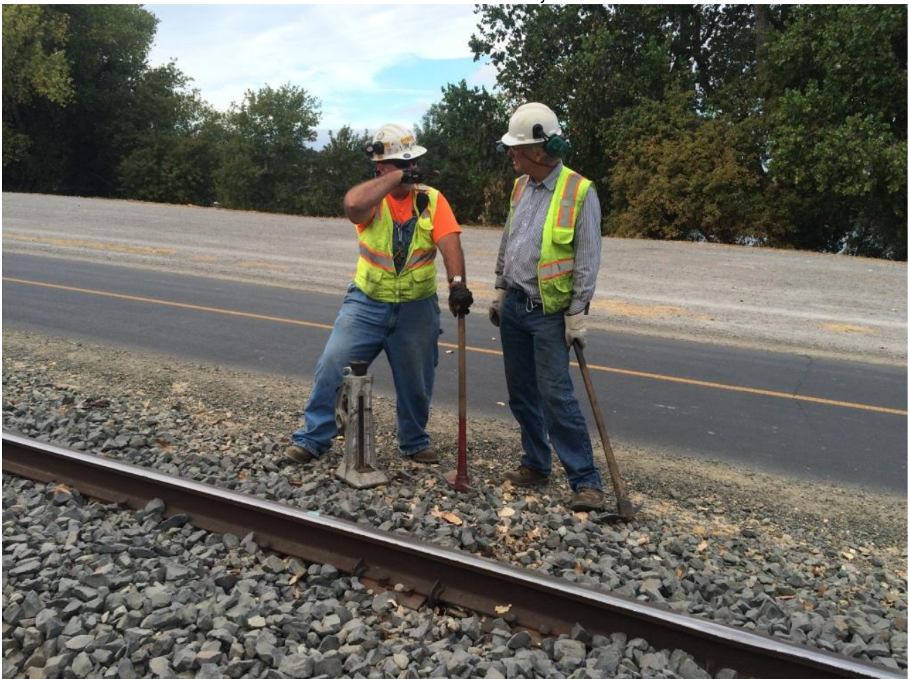
Mike F. demonstrates to Steve, "We're going to raise the track this high..."
