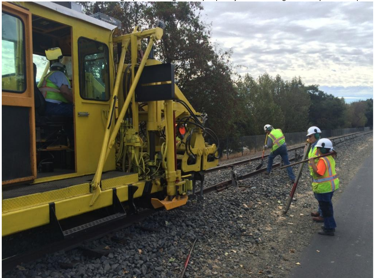
Harry operates the tamper. Steve shifts rock. Pam ready to pull the next jack and Mike W. maintains the track-level
