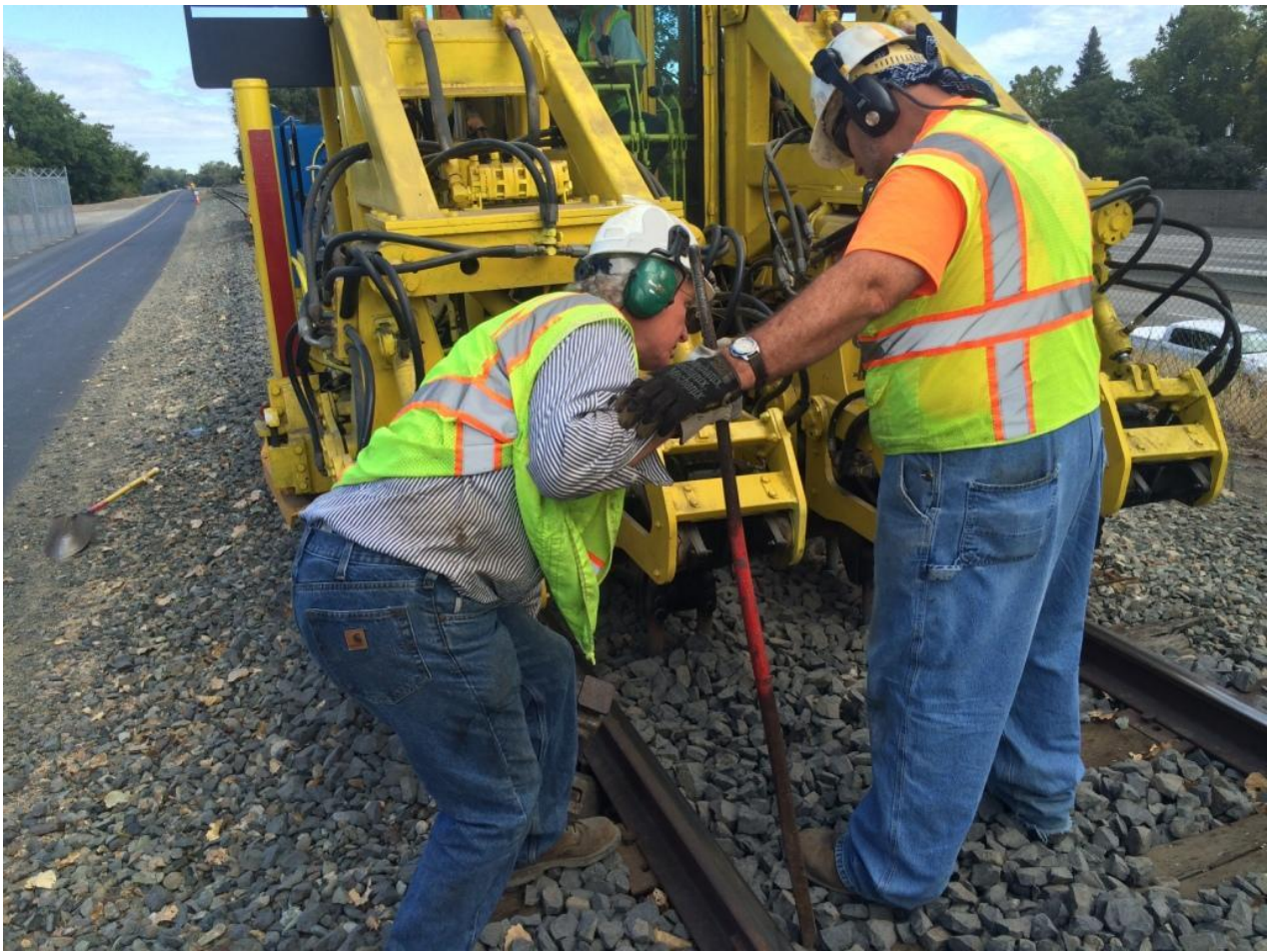
Mike F. offers a helping hand as Steve pulls a jack prior to the tamper tamping that tie
