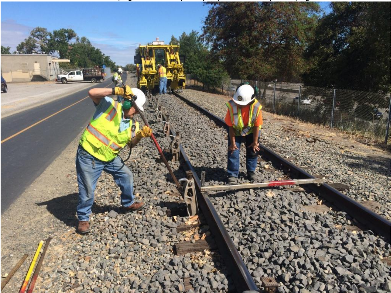
Leap-frogging forward, Mike W. and Pam jack and level the track
