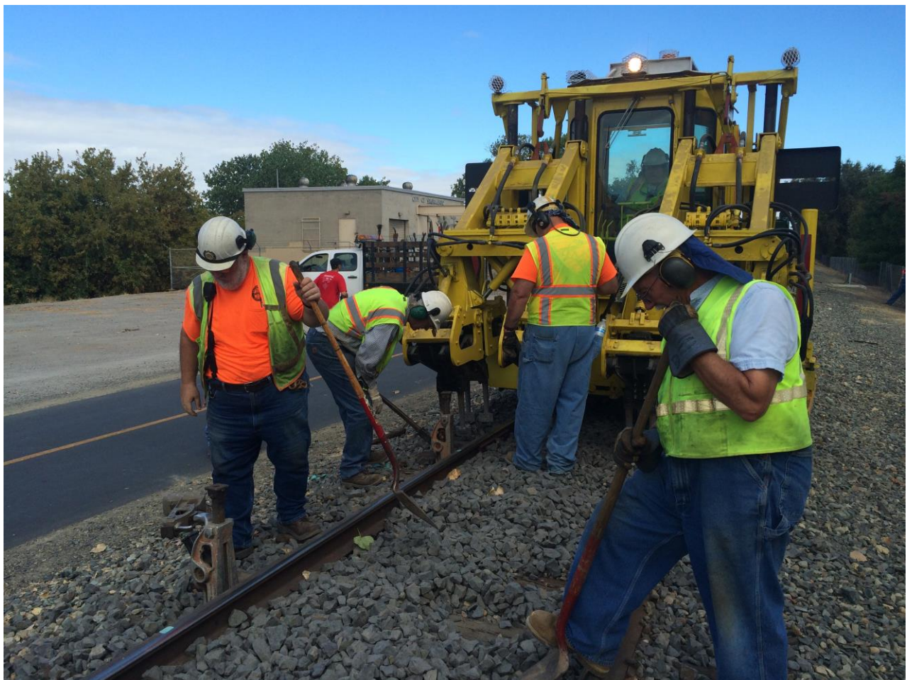
Frank and Clem shift rock into the right place. Steve gets ready to pull a jack as Mike F. guides Harry in the tamper
