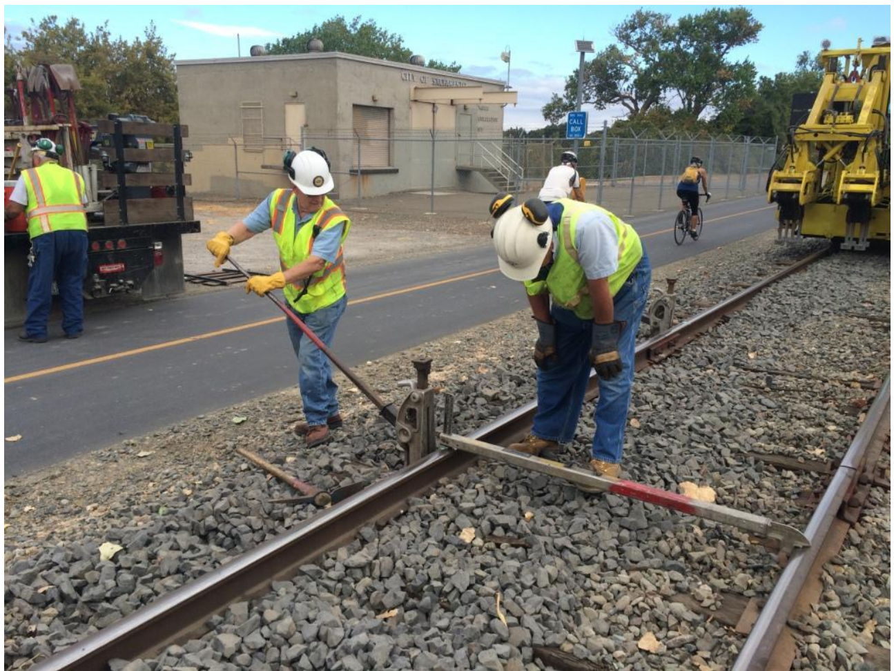
Mike W. jacks the track as Clem checks the level
