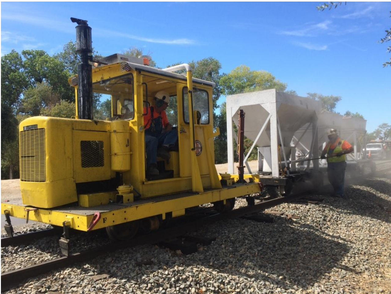
Dave pilots the Kalamazoo as Mike F. drops ballast-rock from the center-dump hopper
