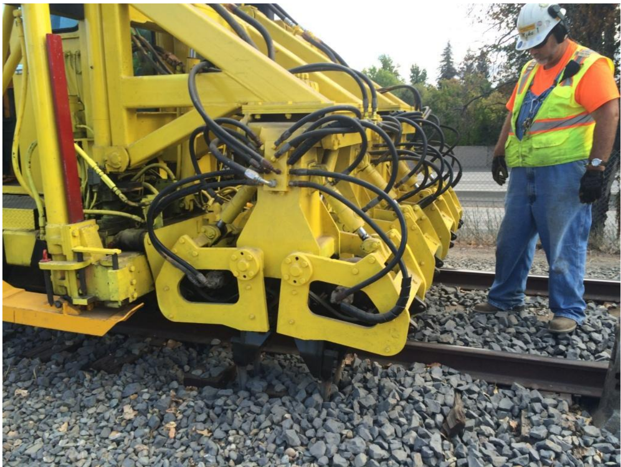
The tamper was working great. The work-heads were descending deeply and the tines were squeezing
